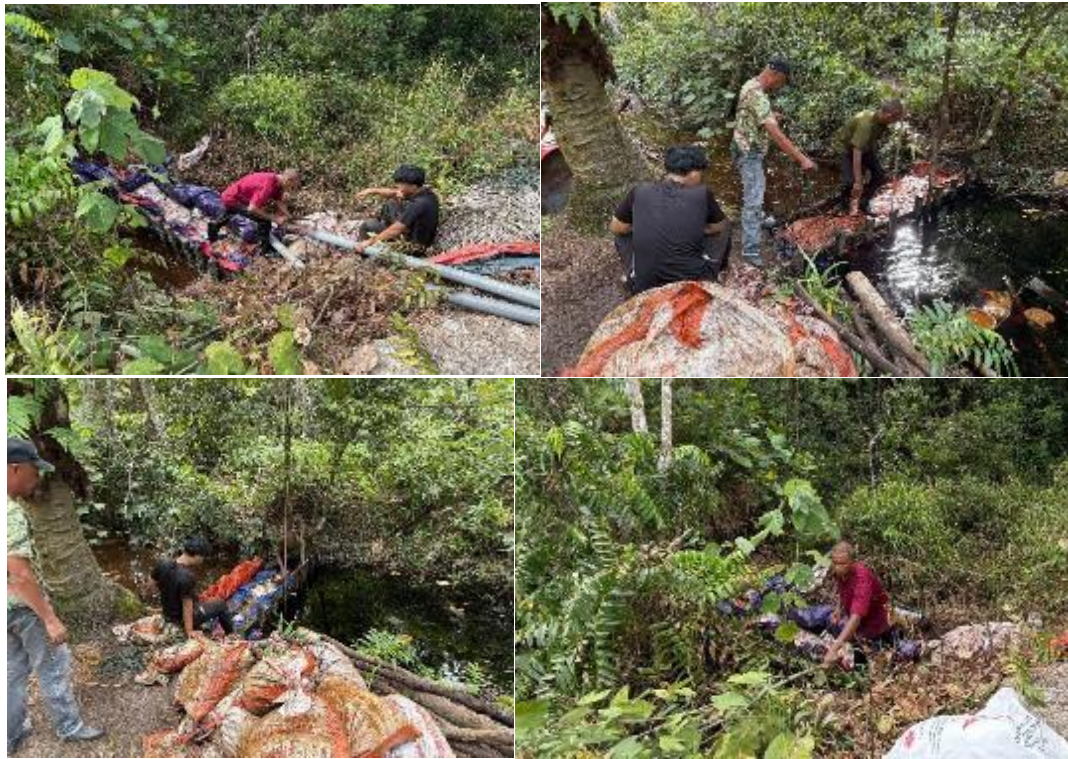
Figure 34. Canal block maintenance undertaken by the KomPAS members
