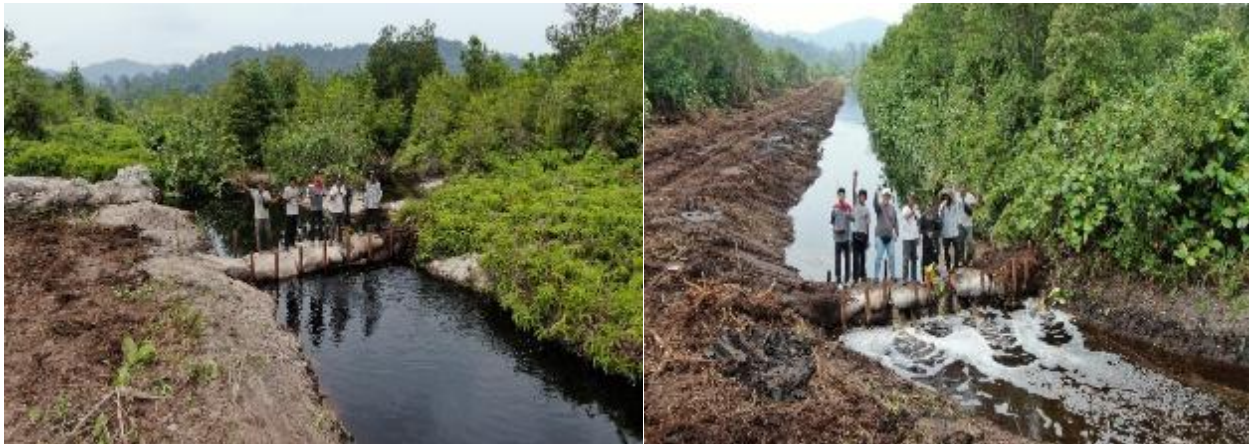
Figure 12. Two canal blocks constructed at Parit Sembilan, Air Papan, Mersing, Johor.
