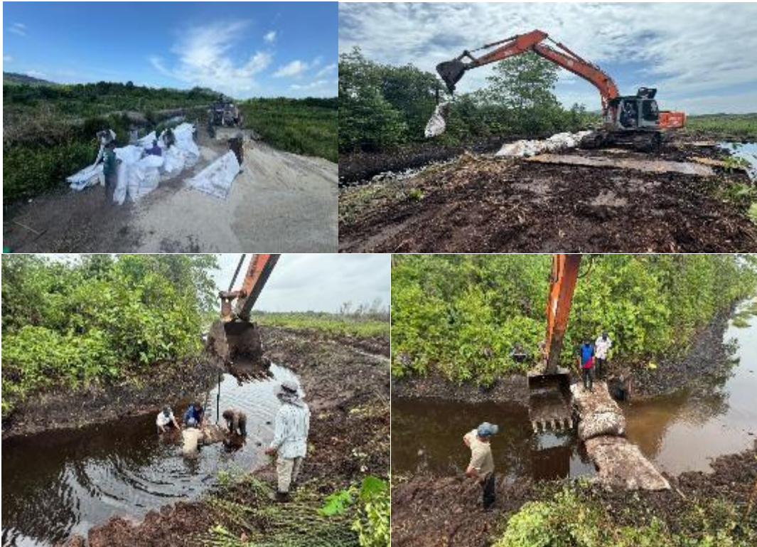
Figure 36. Check dam construction undertaken together with the KomPAS members
